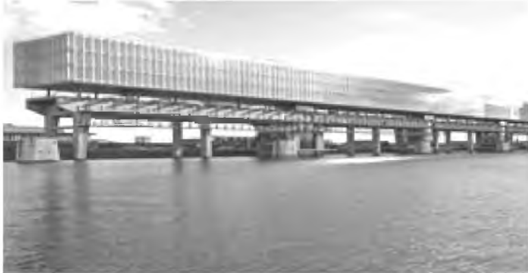
Figure 2. Kraanspoor office in Amsterdam
