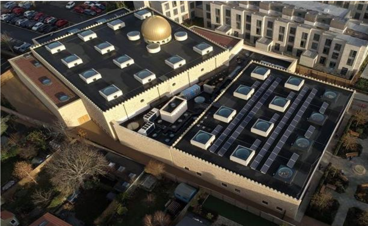
Fig. 5. Central mosque, Cambridge (UK): Placing solar panels on the roof of the mosque [13].
