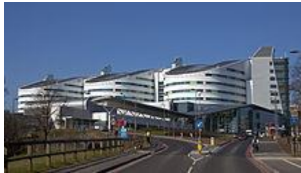
The Queen Elizabeth Hospital Birmingham, a major NHS hospital
