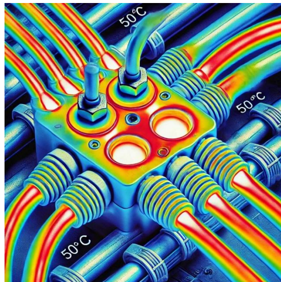
Fig.1. Thermal map of wire connections with excessive heating.
